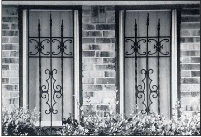
Picket castings #2 and #9 combined with spear point #8206 as a window guard.
