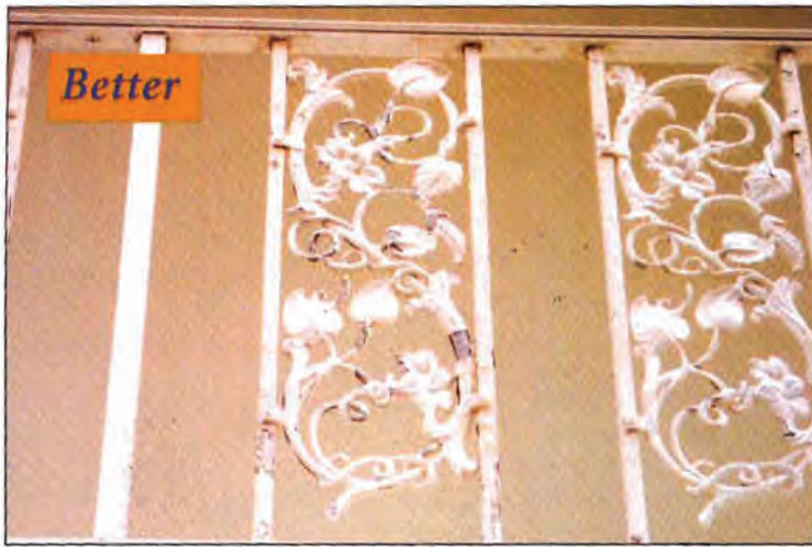
This flower panel in West Palm Beach, FL, shows flaking because of a poor coating job. But its marine grade castings are still shiny and coherent after eight years.
