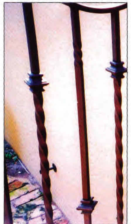
This aluminum rail with marine grade aluminum cast collars also shows a coherent coating in excellent condition after three years on Florida's Intracoastal Waterway.
