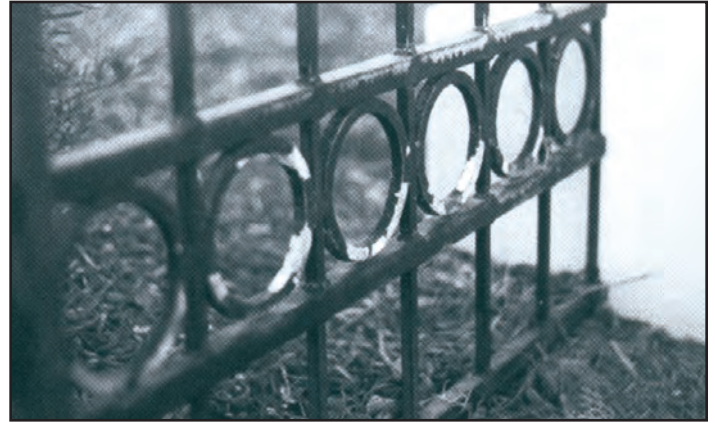
Below and right: White corrosion has deteriorated the powder coating on the floor flange below and on the metal rings of this cast iron gate.
